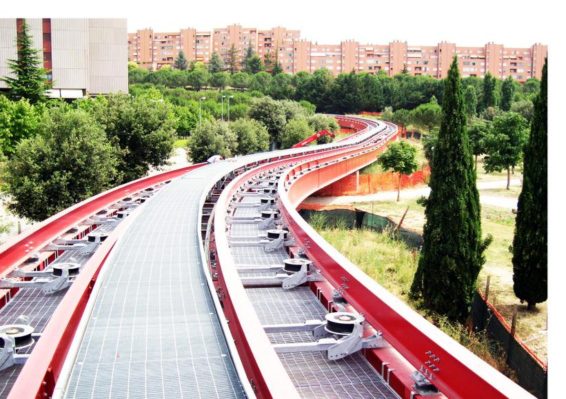
to the rope again. This metro line has been realized, in its elevated parts, with a steel deck made of welded beams with different dimensions, basing on the elevation. The
