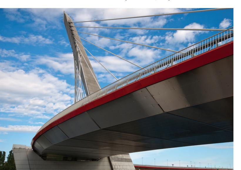
reaches 4.710 tons. The area surrounding the construction site has always remained open to port and road traffic limiting the maneuvering space. It required to assemble the central spans above the dock from a barge and then placed them between the central pillar and temporary towers
